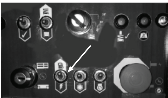
Figure 11.2 - Diesel / Electric Selection Switch
